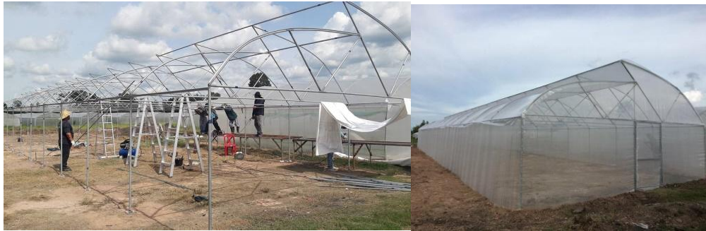
Figure 6 Construction of prototype greenhouses
