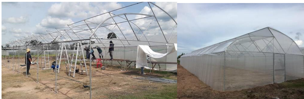
Figure 6 Construction of prototype greenhouses
