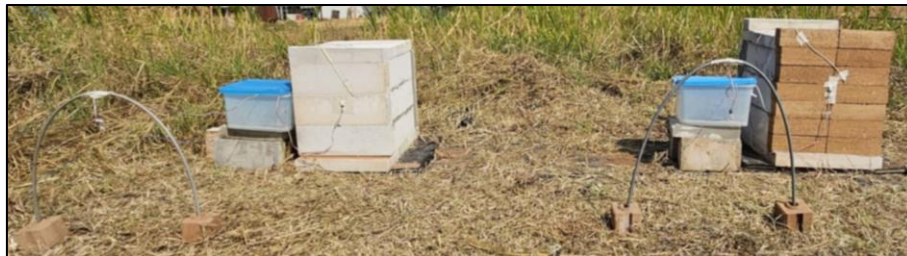
Figure 10. Constructing Box-Shaped Building for Field Testing of Heat Transfer
