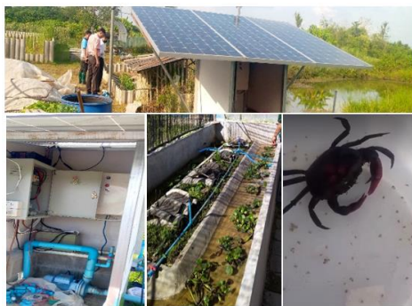
Figure 1. Rice field crab farming worksite in Hankaew district, Hangdong, Chiang Mai, Thailand. (Top) PV module installations, (Bottom): (Left) Commercial MPPT charger in the control cabinet, (Middle) Existing recirculation water system, and (Right) Rice field crab and larvae (small black spots)
