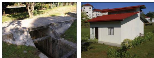
Figure 5. Structures made from OPS concrete. (Left) Footbridge and (Right) Low-cost house (Teo et al. , 2006a)
