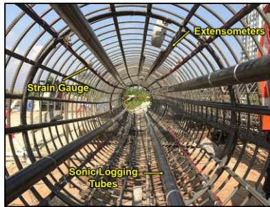
Figure 6. Test pile instrumentation
