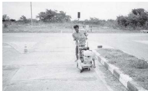
Figure 7. Road cutting of a standard detector
