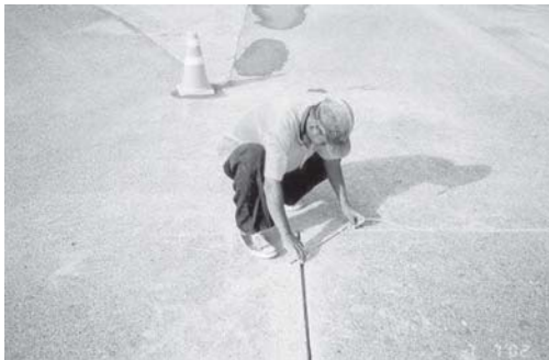
Figure 9. Road cut and wiring around a corner
