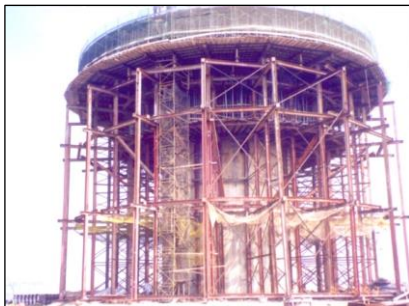
Figure 1. Ground Support: Conventional Scaffolding Systems (Jeng et al. , 2000)
