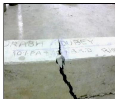
Figure 8. Failure of PCCB
