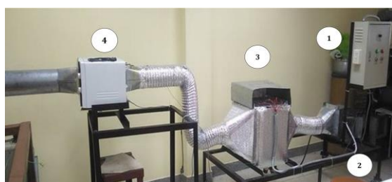
Figure 1. Drying equipment consisting of a system controller (1), a ½-hp blower (2), 8-kW heating box (3), and a drying chamber (4)
