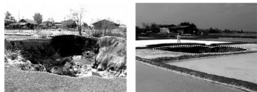
Figure 2. Sinkholes caused by brine pumping in Sakon Nakhon province, northeast of Thailand (Wannakao et al. , 2005)
