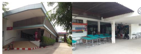
Figure 4. Chakkarat hospital (left) and Chokchai hospital (right)
