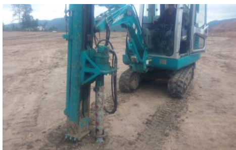
Figure 3. Ground screw pile installation by piling machine
