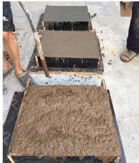
(b) Casting of beam specimens
