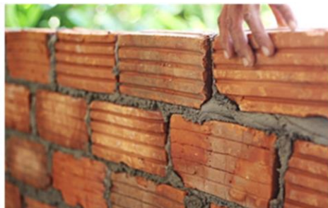
(b) Architectural wall (Haxon Construction and Real Estate, 2018)
