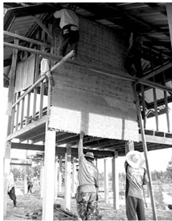
Figure 11. Installation of the woven wall in experimental building
