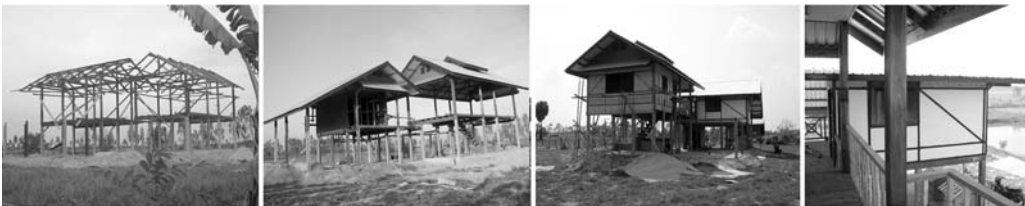
Figure 12. Various phase of experimental dwelling construction: mainframe, covered roof, fixed wall completed floor
