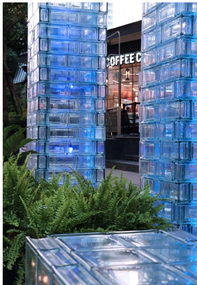
Figure 11. Detail view of glass blocks integrated with vegetation, demonstrating the relationship between material transparency, light diffusion, and vegetation.
