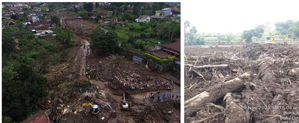
Figure 2 Photograph of flooding in the Kricik River
